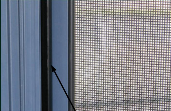
**Step One** Locate spring loaded lock handle. Shown here in black.
