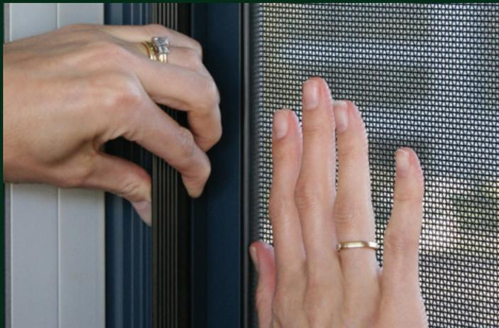
**Step Three** Push escape sash open. The sash should freely swing outward.
