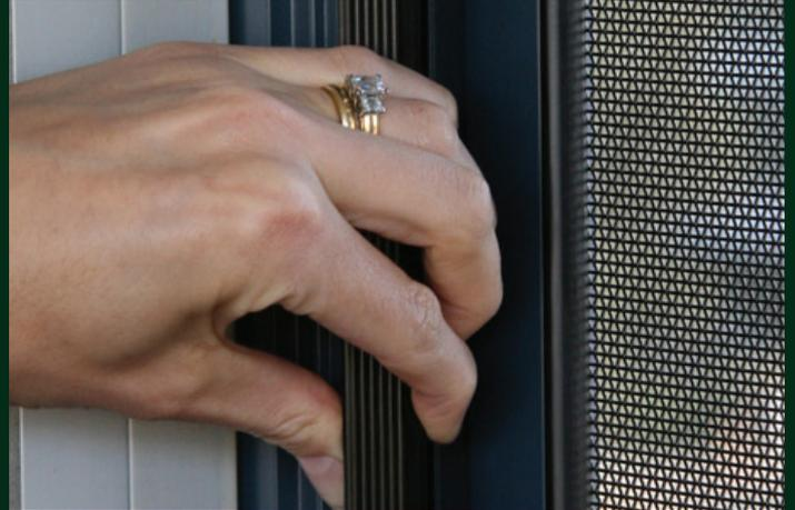
**Step Two** Insert fingers and squeeze handle toward the external frame.
